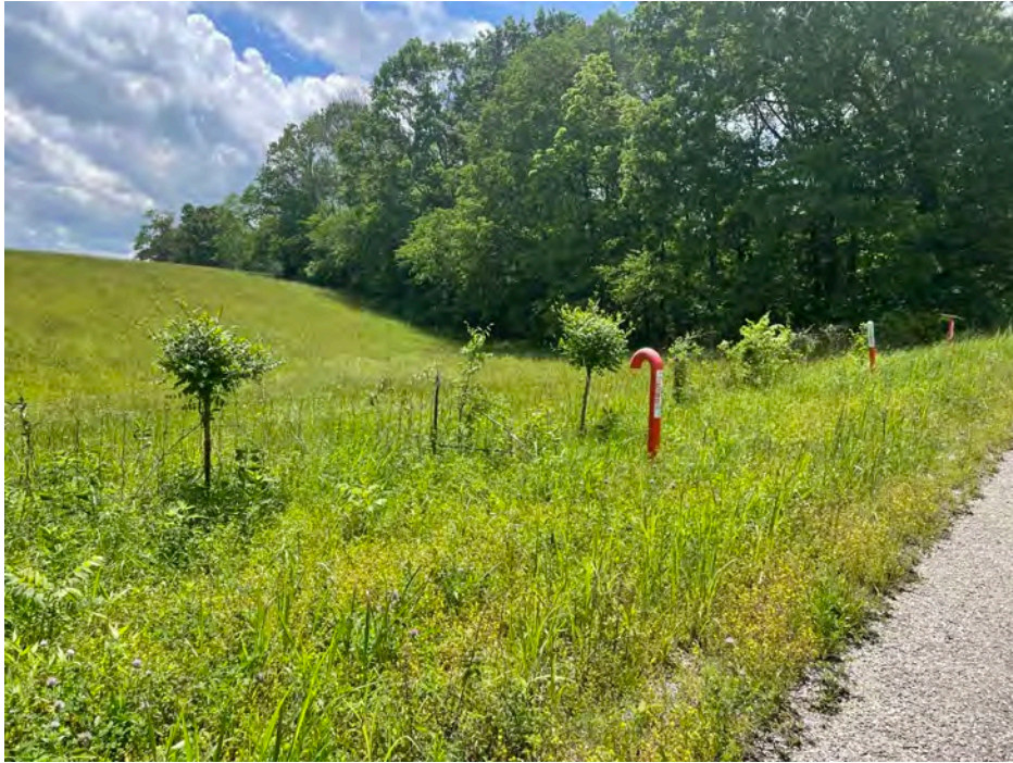
Photograph 5: View of markers for buried natural gas line along the northwest property line.
